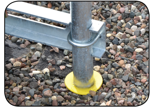
Rail pads protect roof surface.
